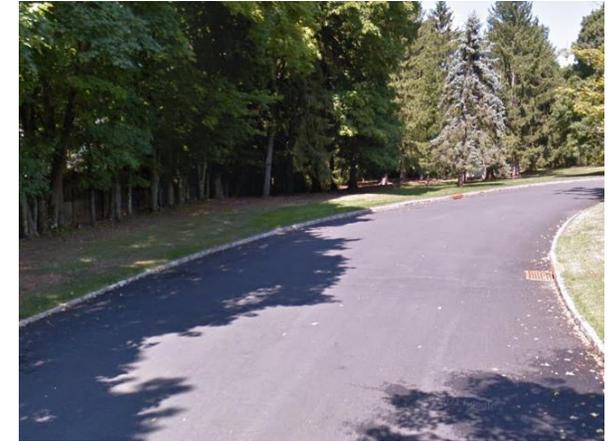
A bioswale can be installed on the corner turn of South Field Drive. This will help with water conveyance down the hill and help prevent erosion alongside the roadway. A preliminary soil assessment suggests that more soil testing would be required before determining the soil's suitability for green infrastructure.
