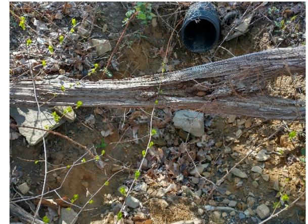
The northwestern section of the pavement can be replaced with a rain garden to intercept stormwater prior to it entering the catch basin. The outfall pipe of the catch basin can be armored with rock to prevent erosion, and the channel downhill of it can be cleared of debris and converted to a bioswale to help promote water infiltration. A preliminary soil assessment suggests that the soils have suitable drainage characteristics for green infrastructure.
